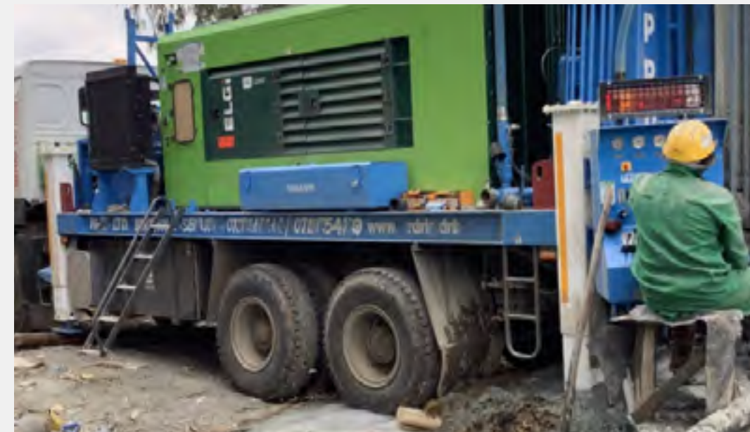
Drilling of borehole
