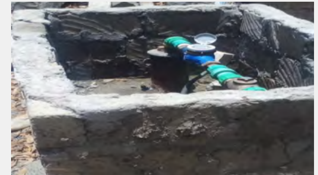
Progress of the borehole to connection to the residence
