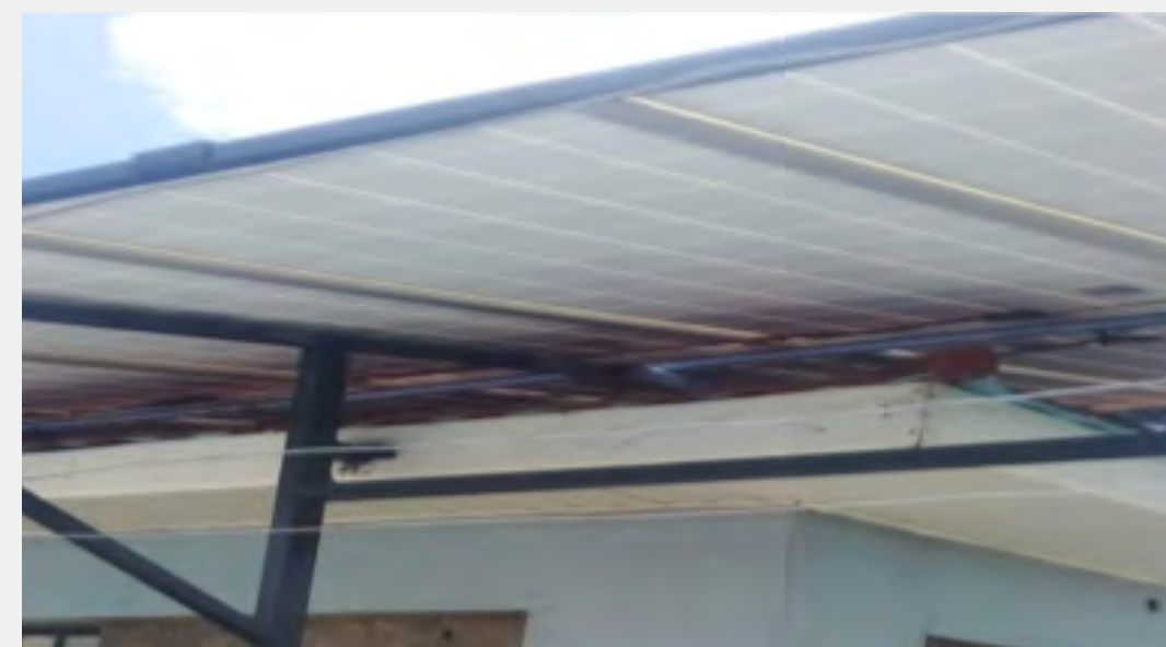
Solar panels installed
