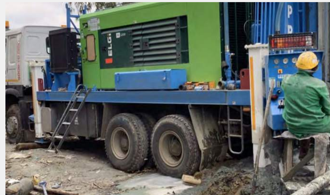
Drilling of borehole
